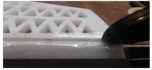
21) Then iron the covering to the leading edge of the alerion. The covering will fill the gap between the wing and the alerion. When you cover the other side, the covering will form a continuous hinge.
